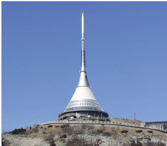
Jizera Mountains, Ještěd - TV tower with revolving restaurant
